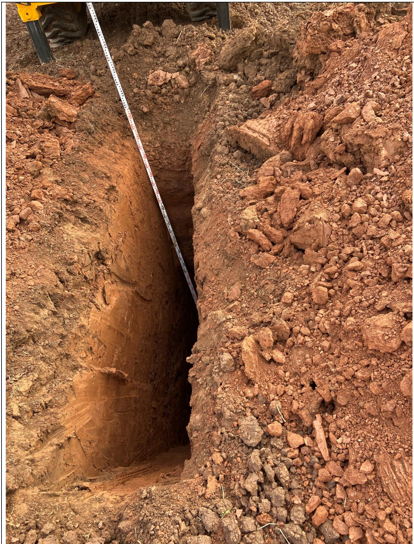
PHOTOGRAPH 3 – TP005 – 0.00m to 4.00m bgl
