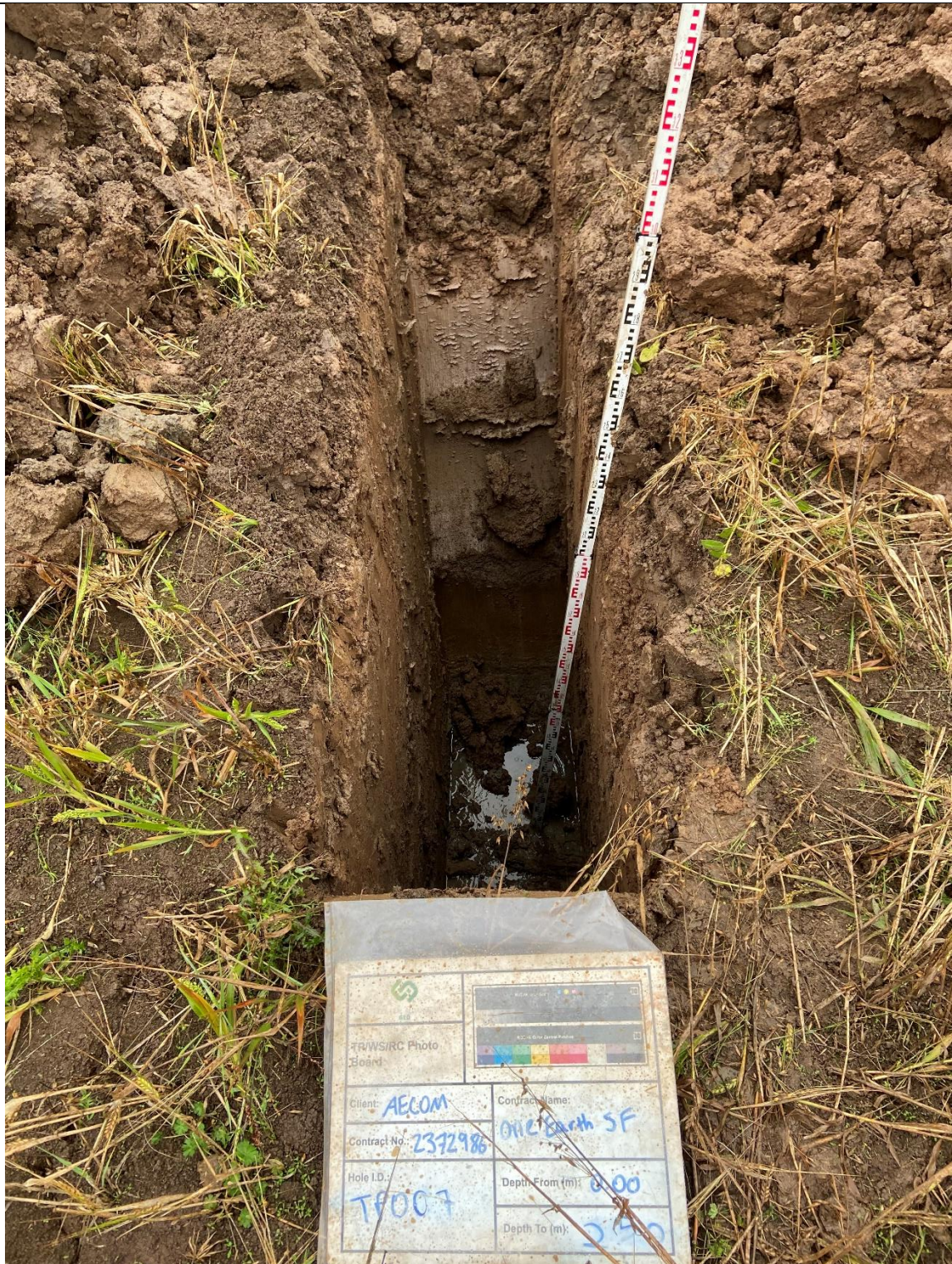
PHOTOGRAPH 1 – TP007 – 0.00m to 2.50m bgl
