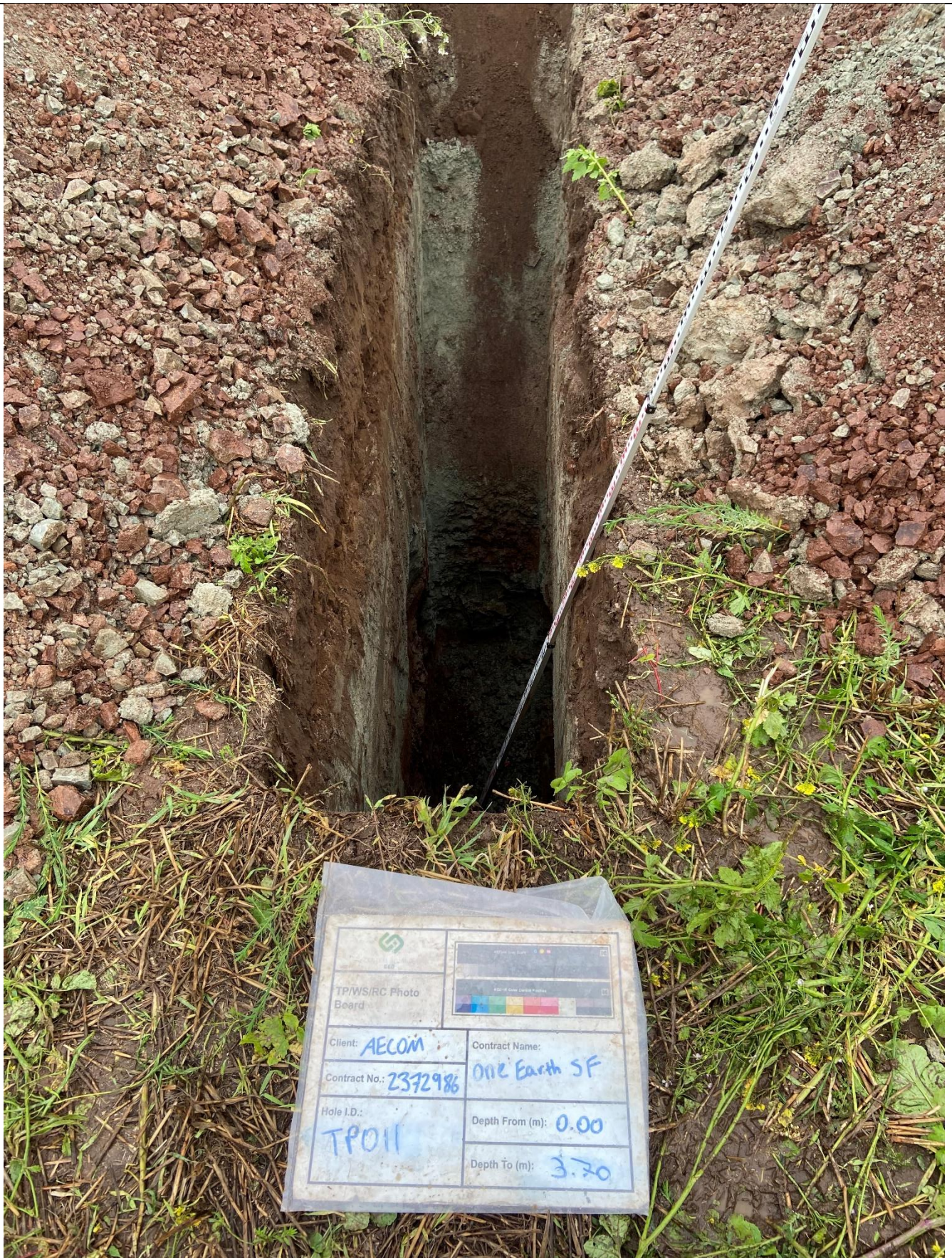
PHOTOGRAPH 2 – TP011 – 0.00m to 3.70m bgl
