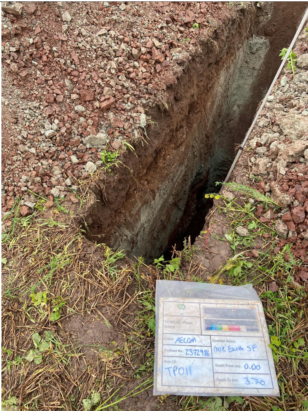
PHOTOGRAPH 3 – TP011 – 0.00m to 3.70m bgl
