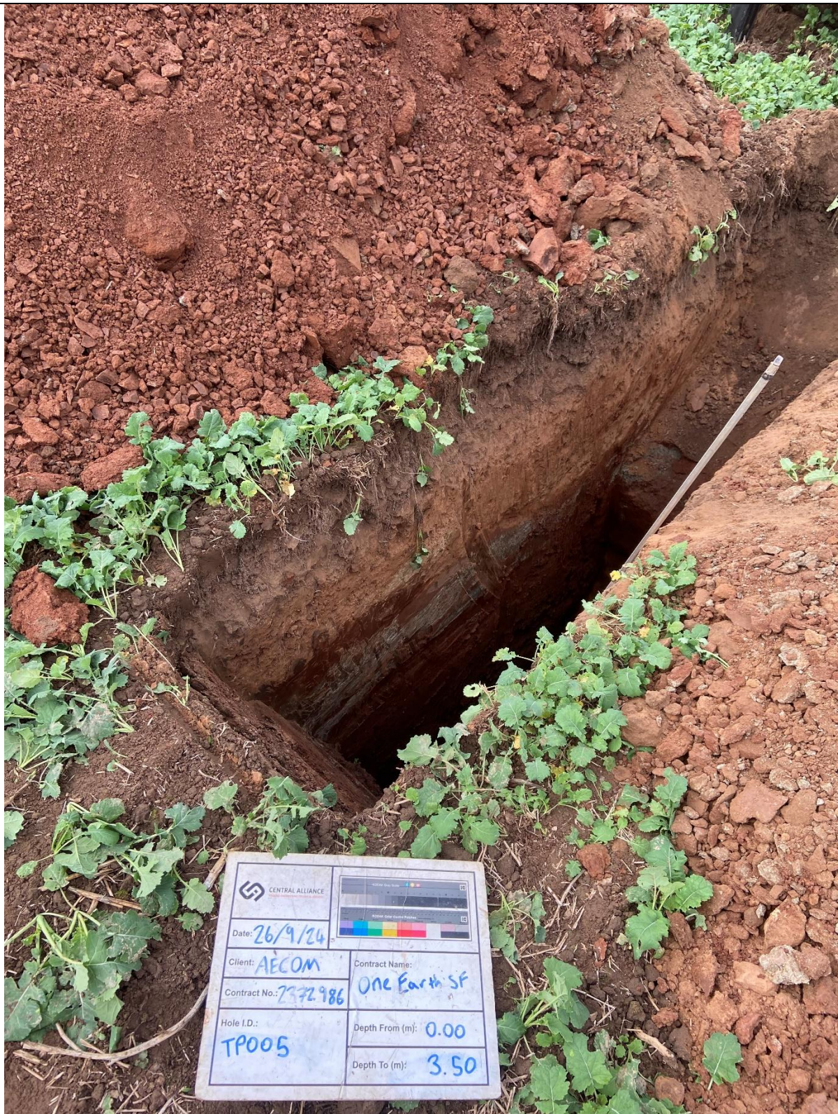
PHOTOGRAPH 3 – TP005 – 0.00m to 3.5m bgl
