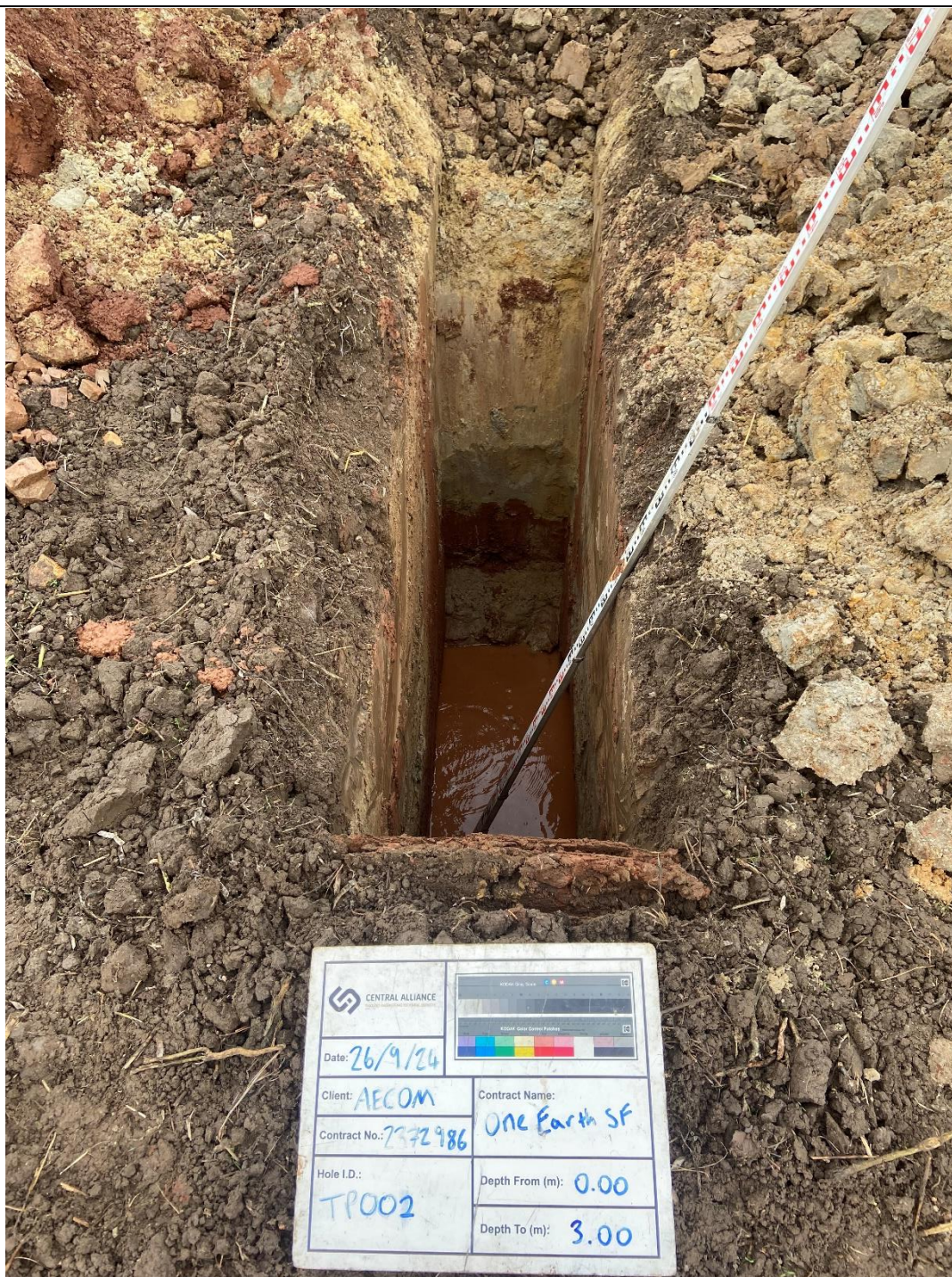
PHOTOGRAPH 2 – TP002 – 0.00m to 3.00m bgl
