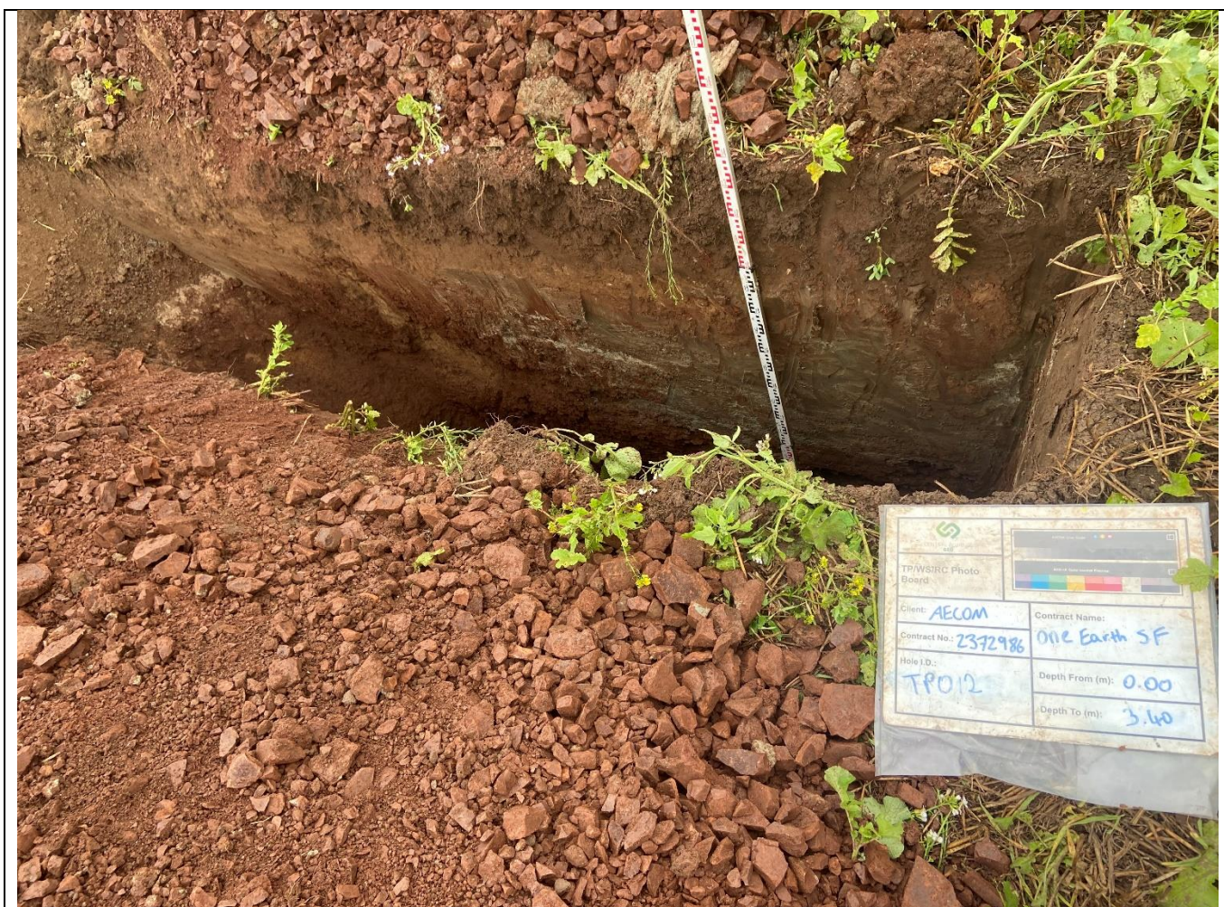
PHOTOGRAPH 1 – TP012 – 0.00m to 3.40m bgl
