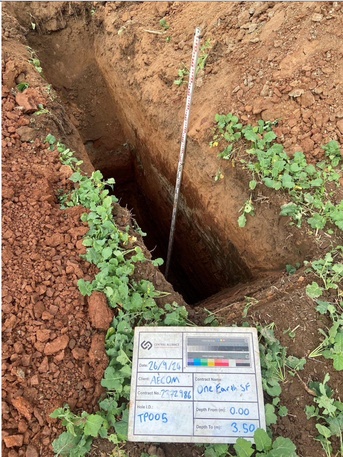
PHOTOGRAPH 1 – TP005 – 0.00m to 3.50m bgl
